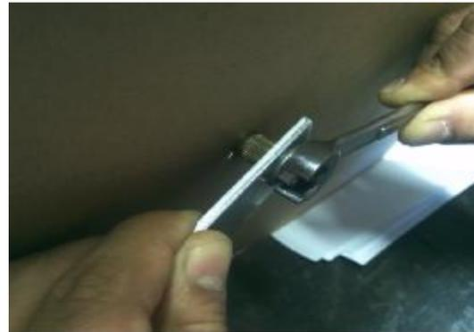
Fig. #5- Shows the tools needed to install the 1/4-20 rivet nut
